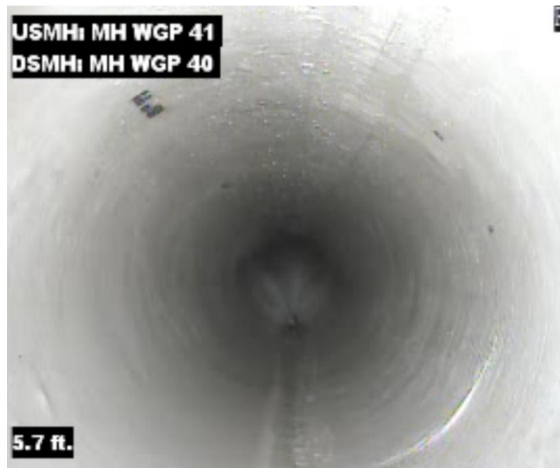
Figure 2 – Same WGP Interceptor Section Post-rehab video with CIPP Liner
